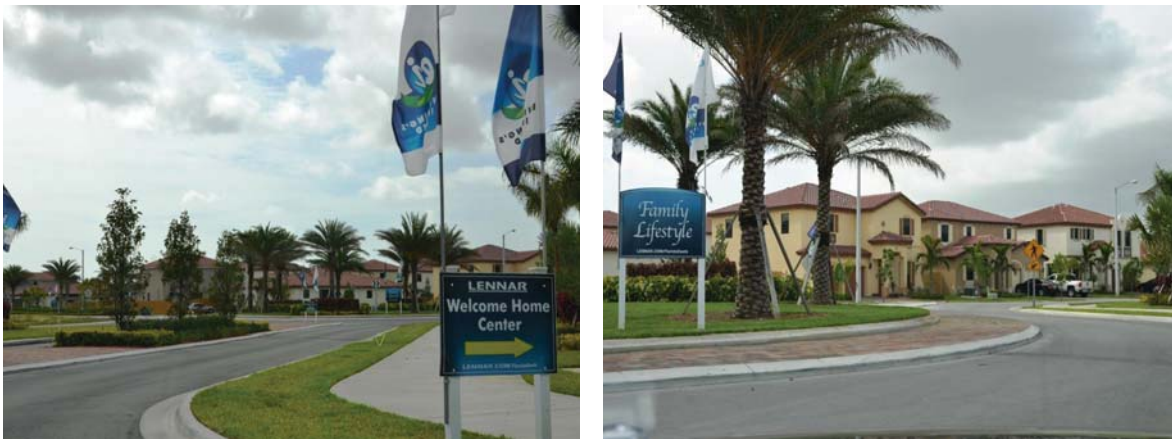
Roads, Drainage, Water, Sewer, Public Park in Assessment Area One (Lennar Area)
