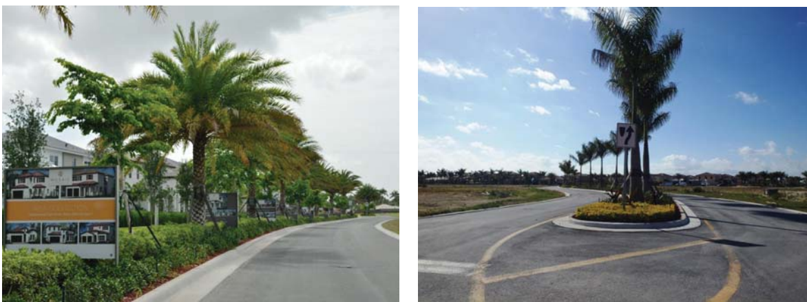
Roads, Drainage, Water, Sewer in Assessment Area Two (Luxcom Area)
